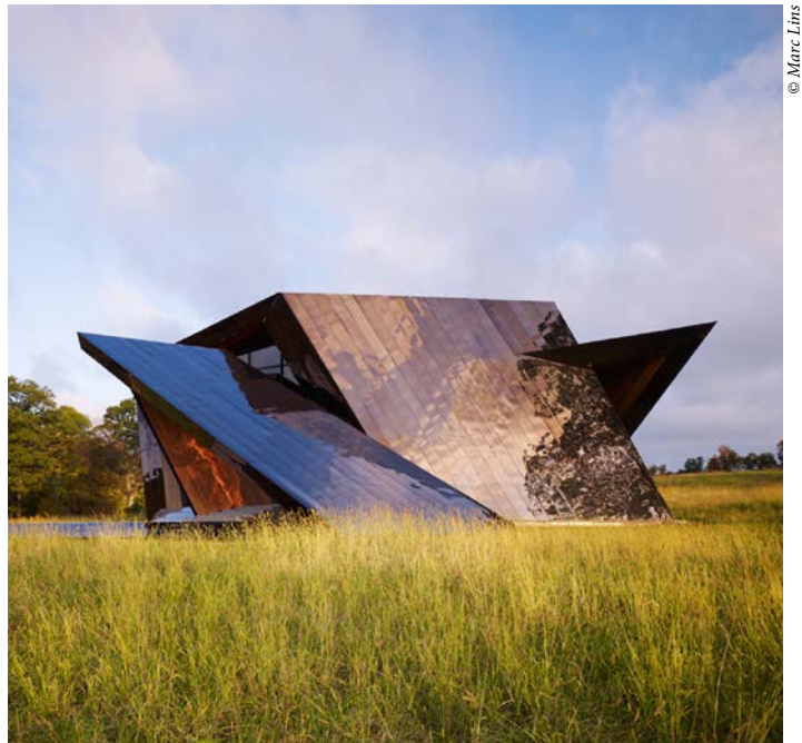
18.36.54 House, Connecticut/ USA
